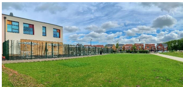
Hartland Avenue entrance next to dining hall
